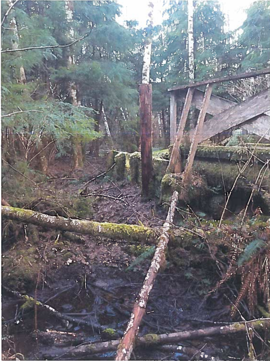
Photo #9 – Fill containment at Bridge #8
