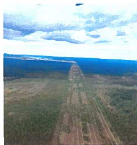
Figure 5. Fuel break linked to transmission line right-of-way
